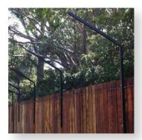
This type of enclosure involves extending an existing fence upwards & inwards. This helps to create an enclosed yard perimeter. This type of enclosure creates very large open spaces, and is an unobtrusive way of keeping your cat contained safely in your yard.
