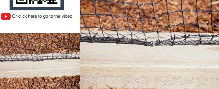
The Black Rope is weaved through the edge of the netting, and then U-Nailed into position.
