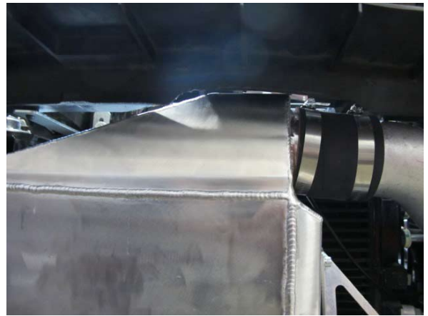
Fig. 9-e: Modified radiator shroud to air/water cooler clearance
