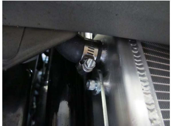
Fig. 8-j: Install short end of 150° molded hose to heat exchanger
