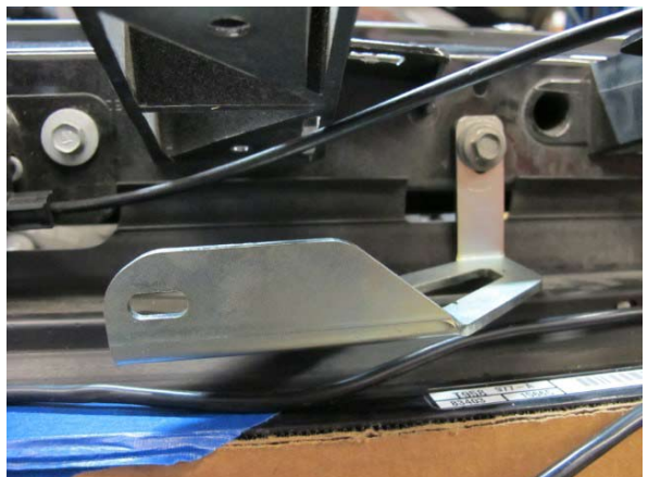
Fig. 6-o: Install upper air/water cooler support bracket
