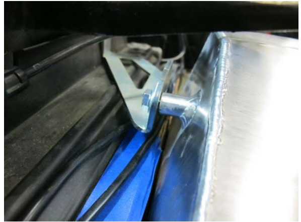
Fig. 6-t: Temporarily secure top side of air/water cooler
